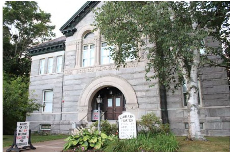
Northfield has used CPA funds to rehabilitate and preserve portions of the Dickinson Memorial Library building.
